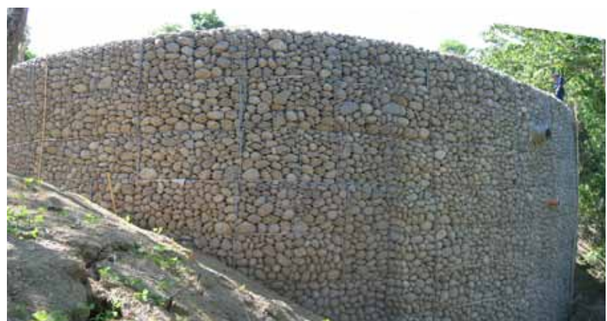
Completed Polyfelt® PEC reinforced gabion wall.
