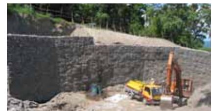
Compaction with 1 tonne walk behind compactor at the MSE wall edge.
